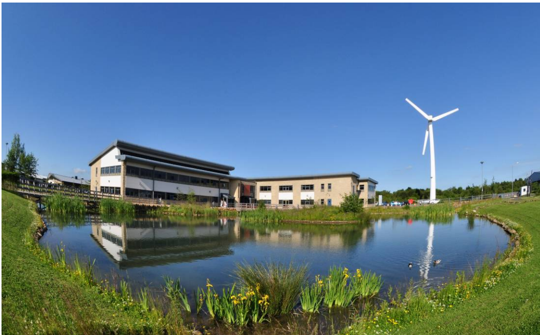
A Vestas V27 turbine at The Greenhouse, Annfield Plain (Image courtesy of The Greenhouse, Groundwork North East)
